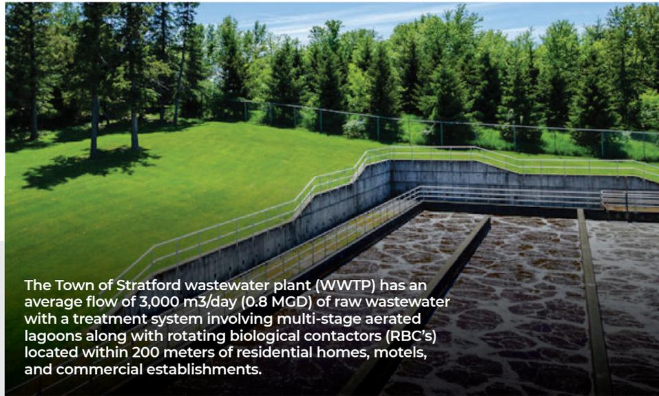
The Town of Stratford wastewater plant (WWTP) has an average flow of 3,000 m<sup>3</sup>/day (0.8 MGD) of raw wastewater with a treatment system involving multi-stage aerated lagoons along with rotating biological contactors (RBC's) located within 200 meters of residential homes, motels, and commercial establishments.
